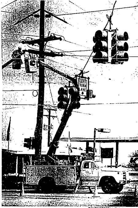
A Detroit Edison crew replaces a cable which had fallen at Grand River and Halsted Road last Thursday afternoon, causing a power outage in some of the Farmington area.
