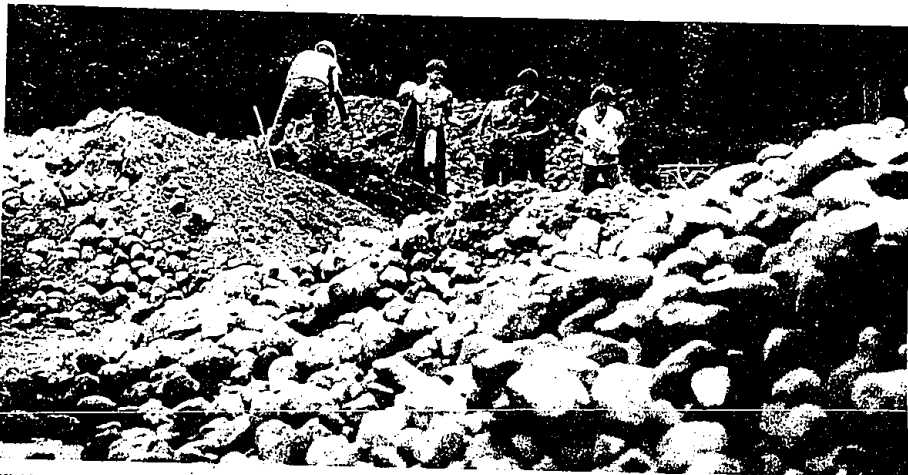
Michigan Youth Job Corps workers choose large rocks which will be inserted into the Upper Rouge River to stabilize the river bank.
