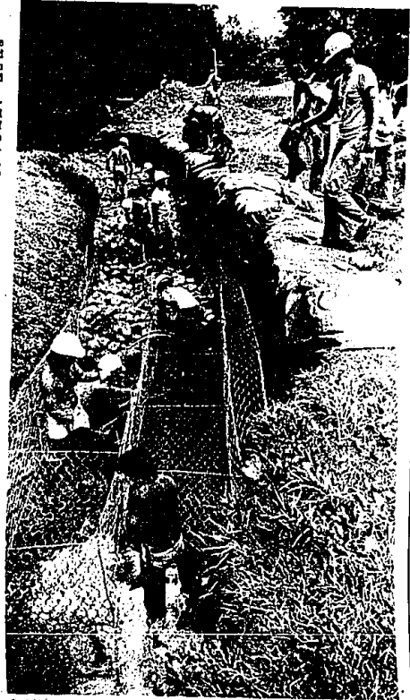
Gabions — wire baskets filled with rocks — are placed in the river to help in erosion control. It is hoped that the project, which began last week, will keep the Upper Rouge River from changing course and causing problems farther downstream.
