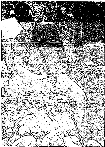
Workman Ed Norwood fashions a gabion — rocks held together with wire mesh — which will help prevent erosion of the stream bank.
