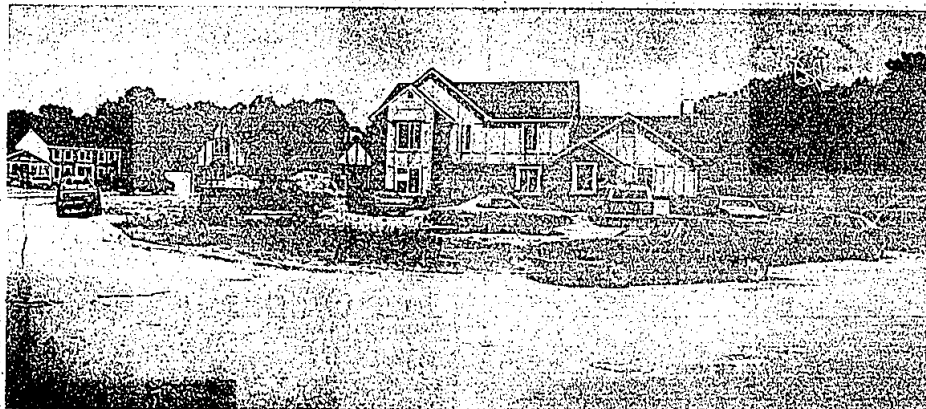
Some of the Homearama homes in the Farmington Brook subdivision receive finishing touches.
