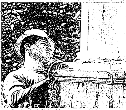
While fellow workers scrape off old paint at the Gov. Warner Mansion, Mike Dyer of Southfield puts on a fresh coat of the cleaning white paint that has long characterized Farmington's historical museum.
