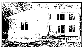
IN TOWN striking brick contemporary under construction, 3 bedrooms plus study, 2-story foyer, Master suite has balcony, Jacuzzi. Birmingham area. $248,000 851-6700
