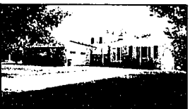
COMMERCE CANAL FRONT. Brick Quad-level with a possible 4th bedroom, 2½ baths, natural fireplace and bar in large family room, walk-out 2 lower levels, attached 2½ car garage and 80 ft. water frontage on wide and deep canal. $114,888 363-8307
