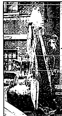
David Kotulski checks his progress on the backhoe as he digs a trench where a curb will be placed. This is the parking lot on the north side of Grand River.
