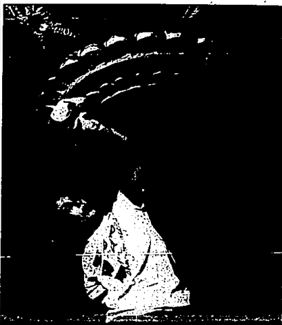
Sonya Winner applies inlaid oil to the stained surface of the ceiling.
