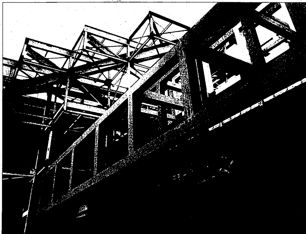
Structural steel detailers produce drawings of every steel connection on commercial buildings. Fabricators make the pieces. Erectors put them
