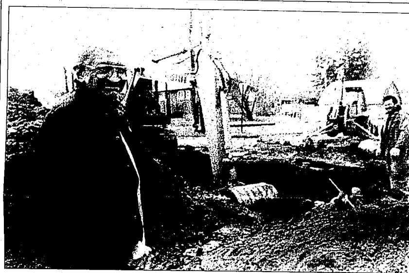
George Roberts, who lives on Ontaga Street, is all smiles as he watches workers improve the water pipes in his southeast Farmington Hills neighborhood. Hopefully, he'll no longer need his emergency bucket of water.
