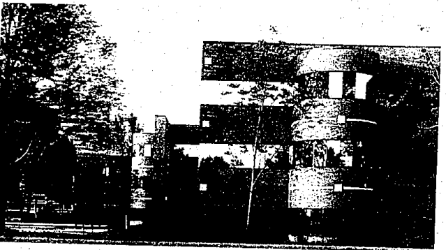
The City Center Office Building features bronze glass in bronze aluminum frames. Four-inch thick limestone inserts set off the brick. Wood, marble, plaster, glass and brass metals were used inside.
