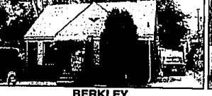
BERKLEY GREAT STARTER HOME . 3 bedroom brick bungalow with natural fireplace, glass block windows, garage with electric and more. $87,900 (806-OB) 548-9100
