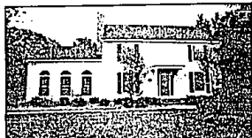
BLOOMFIELD VILLAGE quality new construction by Millcreek. Impressive library, 4 bedrooms including 1st floor master, 2 1/2 baths. Handsome wood trim. Central air, 3 car garage. Home is ready to move into. $417,500. (644-6300)
