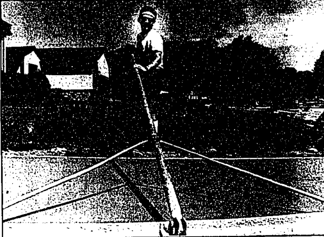
Smoothing it out: Jerry Schieweck of Future Construction puts the finishing touches on new concrete work in the Kendallwood subdivision.
