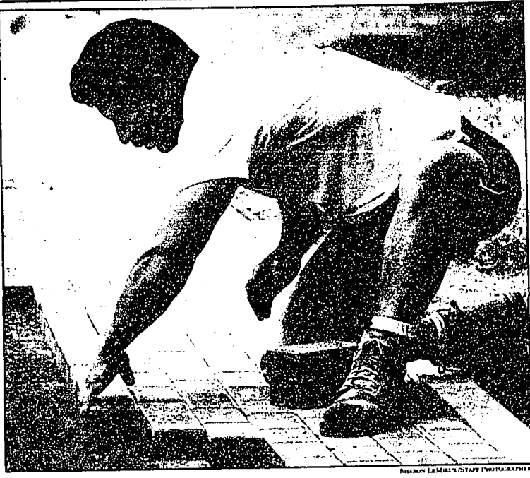
Fitting the bricks: Scott Bruglio of Bruglio Landscaping of Warren lays the brick pathway in front of historic homes on Farmington Road.
