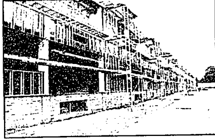
Hip and tuck: North Farmington High is receiving a new facade as well as an expanded cafeteria and media center. The school was built in 1961.
