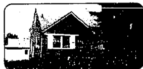
BERKLEY BUNGALOW - Three bedroom, garage, water-proofed basement, new windows - all for only $103,900! (76ELL) 280-4777
