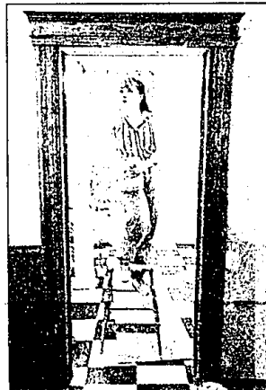
Restoring: Valerie Skowronek paints the trim around the doorway of a bathroom just outside the kitchen. In the foreground you can see the detailed wood trim and original wainscoting.
