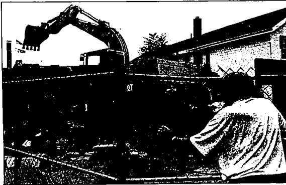
John Cowley watches crews demolish his Old Village Inn. The totally reconstructed Inn is scheduled to open in late February, just in time for St. Patrick's Day.
