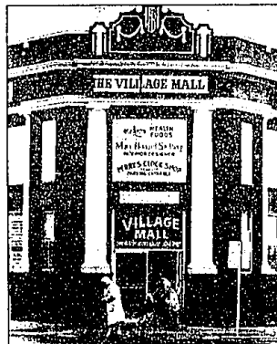
A dated photograph of the exterior of the Village Mall shows how its many unique features have stood the test of time. A recent makeover of a creamy limestone finish with four complementary shades gives the Village Mall a fresh look today.
