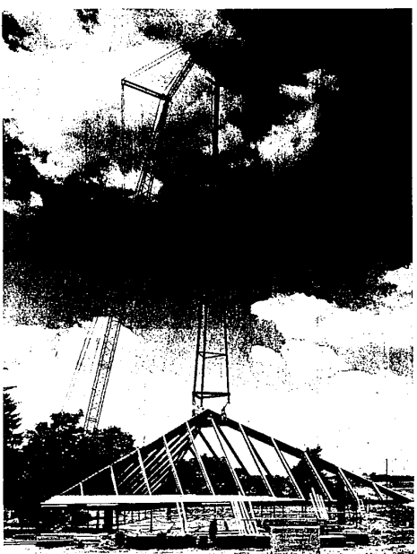
A STEEL TOWER that is bound to become a landmark in Farmington was lifted into place atop the frame of the new University Hills Church at Farmington Road and the I-696 Freeway last week. The tower weighs 6 1/2 tons and will rise 165 feet into the air. It was assembled on the ground before the huge crane gently lowered it to the peak of the triangular-shaped church building. The church, being constructed by C.H. Haberkorn & Co., Orchard Lake general contractor, is due for completion in mid-October.
