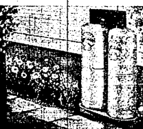
When Shellane is installed at your home, two cylinders are placed in some inconspicuous place outside the house and covered with a neat canopy. Through concealed copper tubes, the gas is then piped directly to your range, refrigerator, or water heater. When one cylinder is exhausted, we replace it promptly upon your order.
