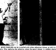
WOOD PANELING can be installed with either adhesives (shown at left) or with nails. After applying the adhesive, place the panel (shown in middle), exerting a steady pressure at all contact points. It is advisable to beat the panel lightly with a soft rubber mallet, or harmer and a padded block, to insure good contact. Finish off the new wall with hardwood moldings, first drilling the nail holes with a drill slightly smaller in size than the nail.
