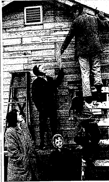
David Byrne, age 11, hands up a board to father Francis Byrne as Mrs. Richard and wife Grace look on. Young Robert Byrne, 5, is more interested in the camera. The Byrne family, burned out of their home at 23166 Springbrook last Thursday morning, is busily engaged in preparing a house for occupancy.
