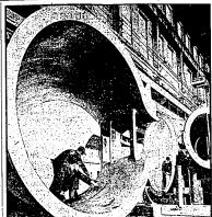
FOR HUNGRY HORSE POWER — These large spiral casing sections are part of one of the four 105,000-horsepower turbines being built for the Bureau of Reclamation's Hungry Horse Dam power plant at Hungry Horse, Mont. Each easing it so large that it is being manufactured in four sections. The four thinese will harness the waters of the South Feed. The four thinese will have been considered the four-section between the Facilite Northwest.
