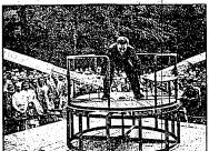
"FLYING" LOW—Using elbow grease instead of a motor, Dr. Fritz Bruns of Herford, Germany, solved the post-war ban on building attrobrae vehicles with this hand-pumped contraption which whizzes around instead of up. The "flying" apparatus has flapping, flexible wings attached to a merry-go-round-like construction and whirls at a speed of about 45 MFH.
