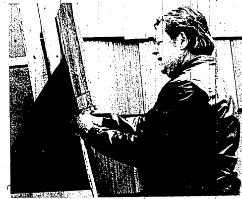
HARRY WALLACE puts up some new siding on the VFW addition.
