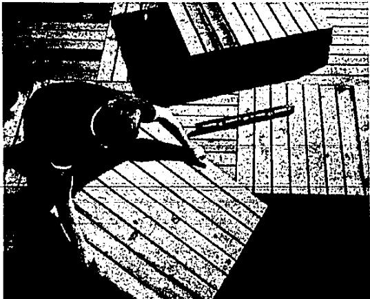
ALL IN A WEEK-END, you can build an exciting outdoor living area. Place three-foot modules of two by four-inch wood in alternating directions over bed of sand and gravel to form parquet-pattern deck. Wood in direct contact with ground should be preservative-treated.
