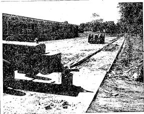
SIDEWALK FORMS were completed the latter part of last week-at the Shiawassee School site and everything was made ready for the pouring of concrete following the long Labor Day week end. The sidewalk will be extended yet ward beyond the school boundary and will just in with the existing sidewalk along the south side.
