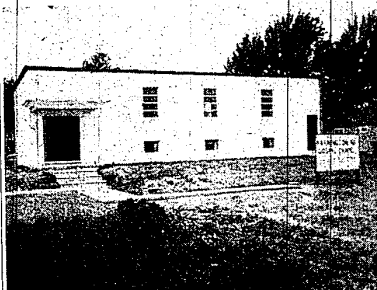
Exterior view of new Chapel at Farmington Road and Kirby Street.
