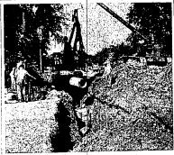
ANOTHER LINK is added to the Farmington Interceptor Swer as workmen continue to push for an early completion of the City project. This section of main, being installed on Nine Mile Road at the intersection of Hanes, is only two blocks from the Farmington City Limits. In the meantime, additional links are being connected on Shiawassen ear find, and the state of the st
