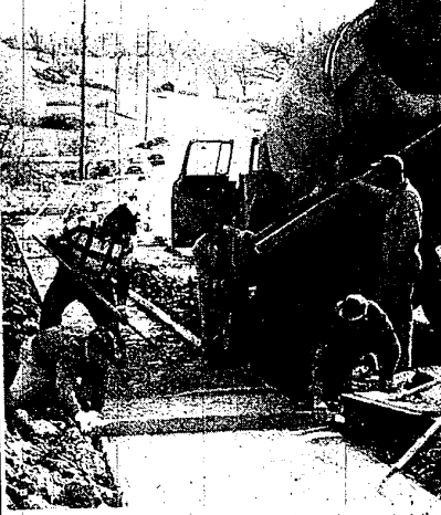
SIDEWALKS ALONG Shiawassee were being laid last week, and this, in an effort by the city to complete the work before winter sets in.
