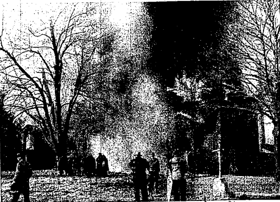
OLD BOYS REPUBLIC was burned out last Sunday as a preliminary to knocking down the remaining walls and clearing the 93-acre tract.
