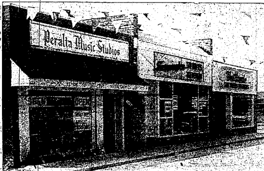
SHOWN ABOVE are the three most recently opened stores in the Westbrooke Shopping Center. Peralta Music Studios, on the left, and Westbrooke Children's
