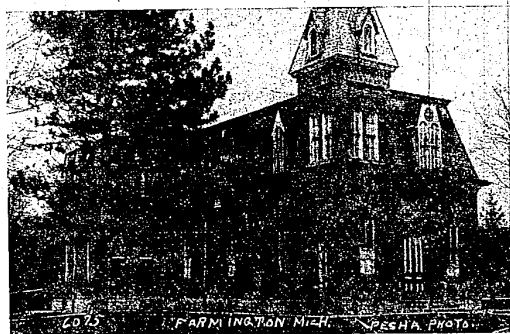
A PHOTOGRAPHER by the name of Pesha took this shot sometime after 1914. The back portion of the Town Hall was added that year. Note the third entrance, unused today, on the Grand River side. The detail of the original was carried out exactly on the addition, even
