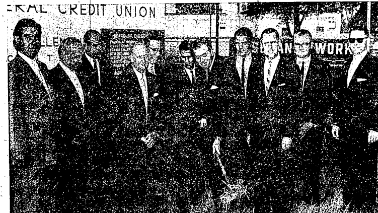
GROUND BREAKING ceremonies for the new Our Lady of Sorrows Parish Credit Union Building were held last Thursday, July 11, on the site of the proposed $50,000 structure, Lakeway Avenue and Grand River. Frank A. Nicholls, president of the Board of Directors, is shown above turning over the first spadeful of dirt as (L to R) architect John Allen, Walter DeMatia, builder Robert J. Pistonetti, Joseph DeNies, Donald J. MacKinnon, Norbert Joanisse, (Nicholls), Robert MacKinnon, Robert Abraham, Charles B. Schwartz and Albert E. Gingell look on with approval.
