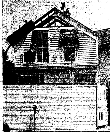
A FAMILIAR OLD BUILDING gave way to progress this past week in the City as the Shoe Repair Shop located on Farmington Road at Grand River underwent remodeling. The 63-year-old building was torn down to provide parking space.
