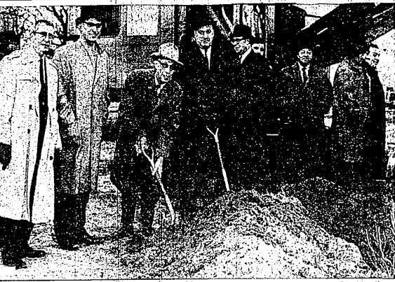
GROUND BREAKING CEREMONIES were held this week for Farmington Township's three million dollar water project and many of the officials, representing some 15 different federal, state and local agencies who cooperated in the long struggle for the much needed facility, were on hand to participate. Pictured above (L to R) are R. J. Alexander, Director of the Oakland County DPW; Delos Hamlin, Chairman of the County Board of Supervisors and the Board of Public Works; two unidentified members of the official party (with shovels); and Township Attorney Joseph T. Brennan with other representatives who turned out to witness the occasion.
