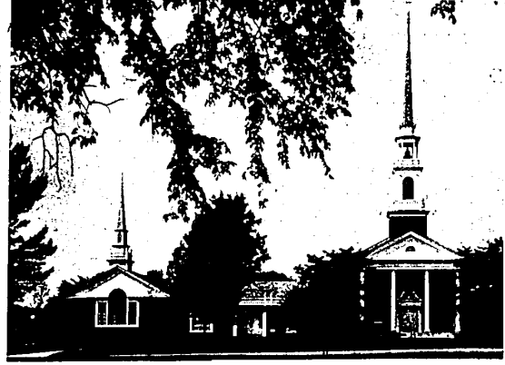
THIS IS A view of the Franklin Community Church, Franklin, which launched the second part of a four-year effort Sunday to pay for a new educational wing. The wing, completed early in 1965, is at the left and also houses a large Fellowship Hall.
