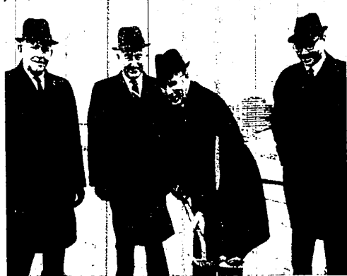
BREAKING GROUND FOR THE 350,000-SQUARE FOOT WAREHOUSE, IN PLYMOUTH TOWNSHIP ON HAGGETT ROAD NEAR JOY ROAD, IS BEING HELD TODAY AT 10:30 A.M. BY PRESIDENT RAY DUTTMER, GENE HOUST, ASSISTANT PRESIDENT, JOSEPH FOY, PRESIDENT OF SPARTAN STORES, INC. OF GRAND RAPIDS. THE NEW FACILITY HAS A TARGET DATE OF EARLY SUMMER AND WILL BE USED TO CARE OF STORES IN SOUTHEASTERN MICHIGAN AND NORTHWESTERN OHIO.
