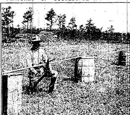
Putting Up the Overhead Irrigation System. Placed on Barrels and Boxes Temporarily While Drilling is Being Done.
