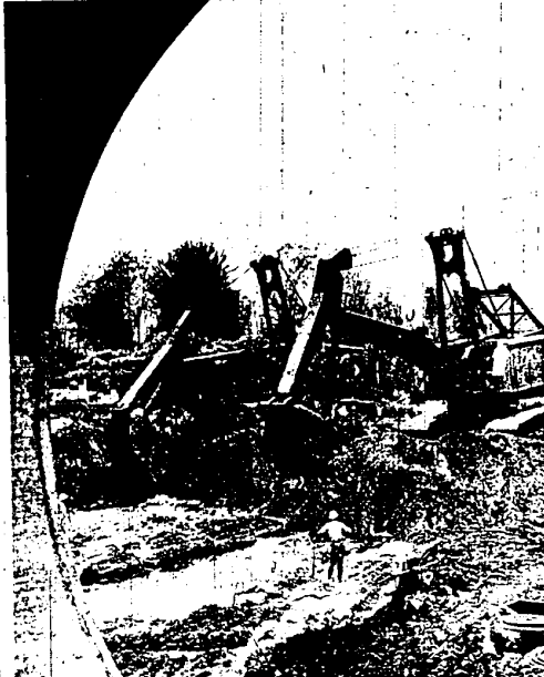
A MILLION DOLLAR storm sewer for the Plymouth-Levan industrial area is under way this summer, with huge construction equipment digging an open cut from Plymouth Road to Schoolcraft Road. Sandy, unpredictable soil conditions and a high water table have harassed workers. Cement sections ten feet in diameter and weighing 23 tons per section are being lowered into place to serve an area of about one square mile. Completion is set for this fall.
