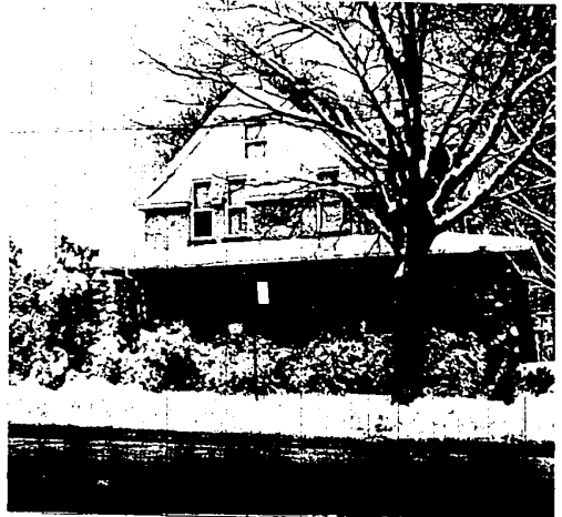
REMODELING WAS DONE on the recently razed house sometime in the early 1900's. The front porch was changed to cover the front of the house and the brick veneer finish was replaced by stucco. In the last two years the house became run-down. The barn had been condemned for three years. The 96-year-old landmark was razed to make use of the land sometime in the future.
