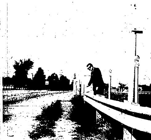
"Here's a glaring example of misuse of a guard rail. A driver going off the road would be forced by the rail into this concrete abutment. The rail should go to the front of the abutment, not into the side." Scene: I-96 in Farmington.
