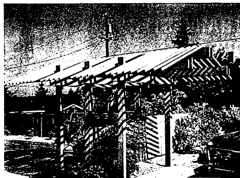
PERGOLA POINTS to entry walk. Fenced front yard needed a gateway to point out the entrance walk, adjoining driveway, and this pergola does the job. Simple structure uses Douglas fir 4x6 posts, 2x6 and 2x8-inch beams and 1x2s on edge for "rafters." Shade-loving plants thrive under pergola's shelter.
