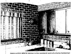
sing only simple household tools. The "bricks" are made of crushed stone nd fiber glass and come in easy - to - install panels.
