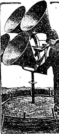
The defenses of Paris against hostile aircraft are well organized. One of the most interesting of the special instruments used is the listening post. It consists of four huge horns which gather up the slightest sound and magnify it by means of a microphone, so that it is impossible for any aircraft to approach unnoticed.
