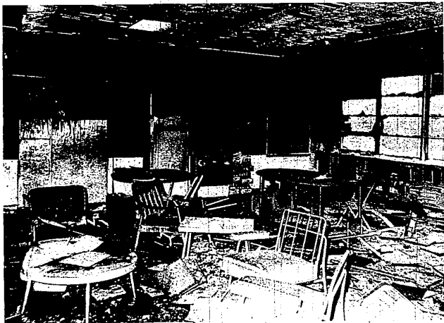
THE TEACHERS' LOUNGE was one of the four rooms severely damaged by the blaze.
