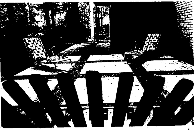
THE ATTRACTIVE PATIO at the Allen Ansell home on La Muro Rd. was a "do-it-yourself" project. Four-foot square cement slabs are surrounded by a bed of grey crushed stone with railroad ties providing an edge to hold the gravel. The contrast in textures is very pleasing and the large cement slabs provide a firm base for chair and table legs.
