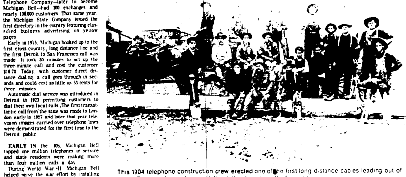
This 1904 telephone construction crew erected one of the first long distance cables leading out of Detroit. The well-dressed man at left with the shovel was the foreman.
