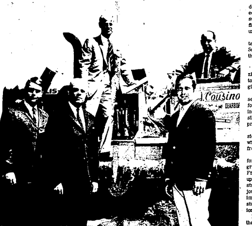
GROUND BREAKING - Ground breaking ceremonies were held last week by A.J. Segal & Sons Contractors, Inc. in the Farmington Industrial Subdivision. Shown from left are Jim Garrison, Dell Garrison, George Segal, Robert Segal, and Tony Asher. (Evert photo)
